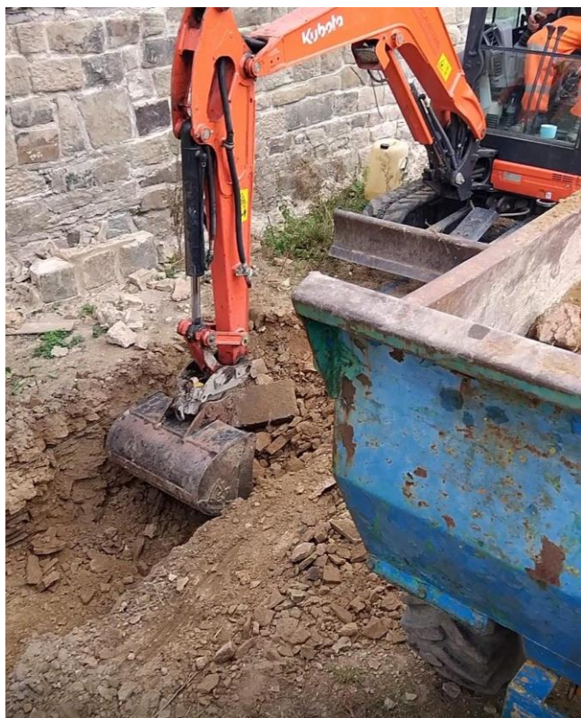
FOUNDATION EXCAVATIONS.
