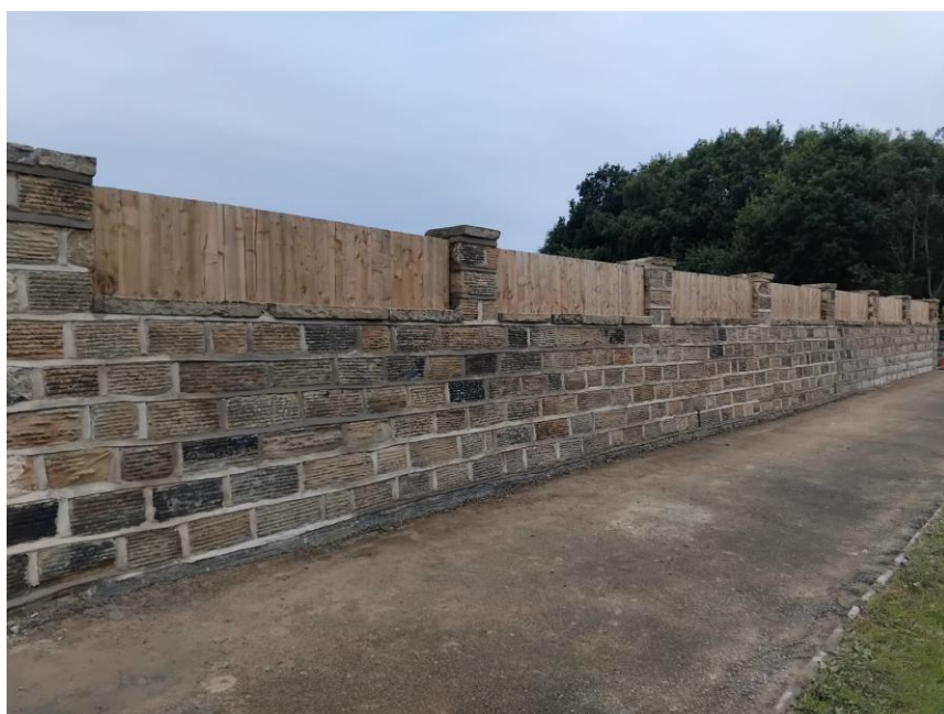
COMPLETED BOUNDARY WALL.
