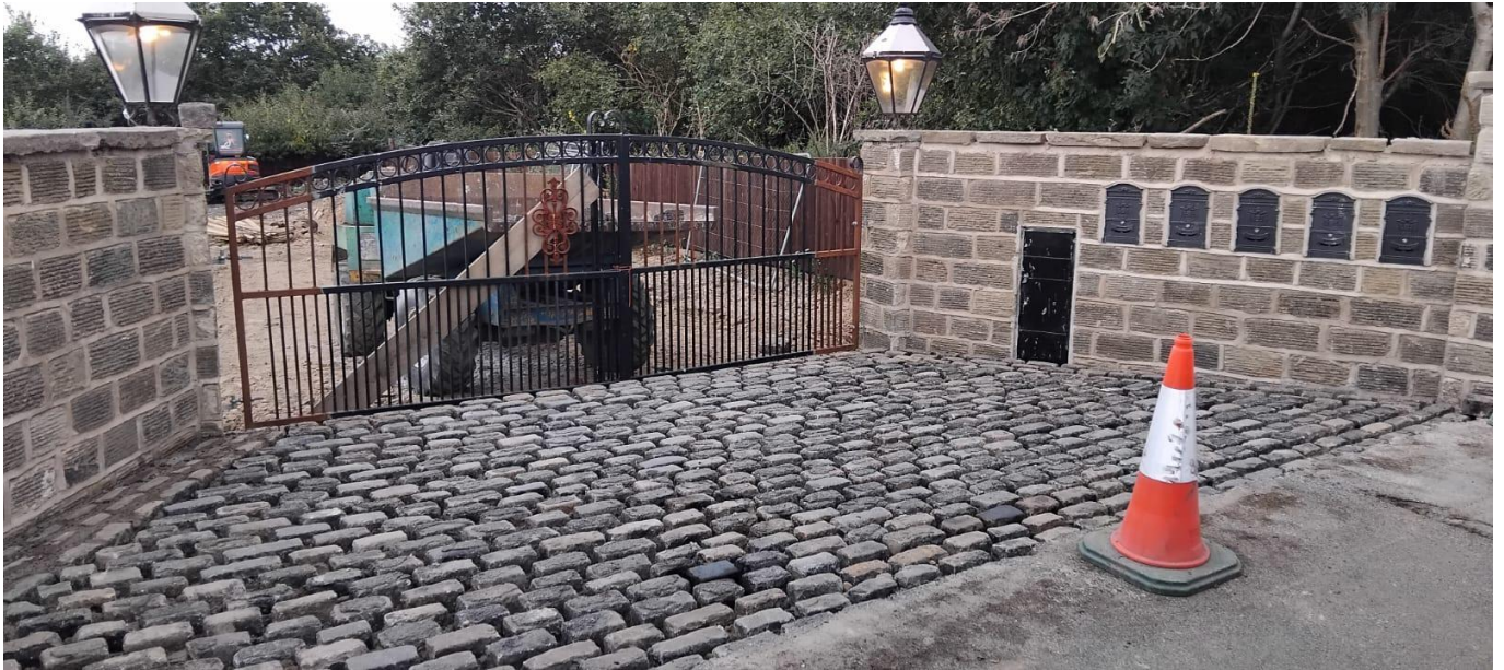
COMPLETED SITE ENTRANCE/ACCESS CROSSOVER
