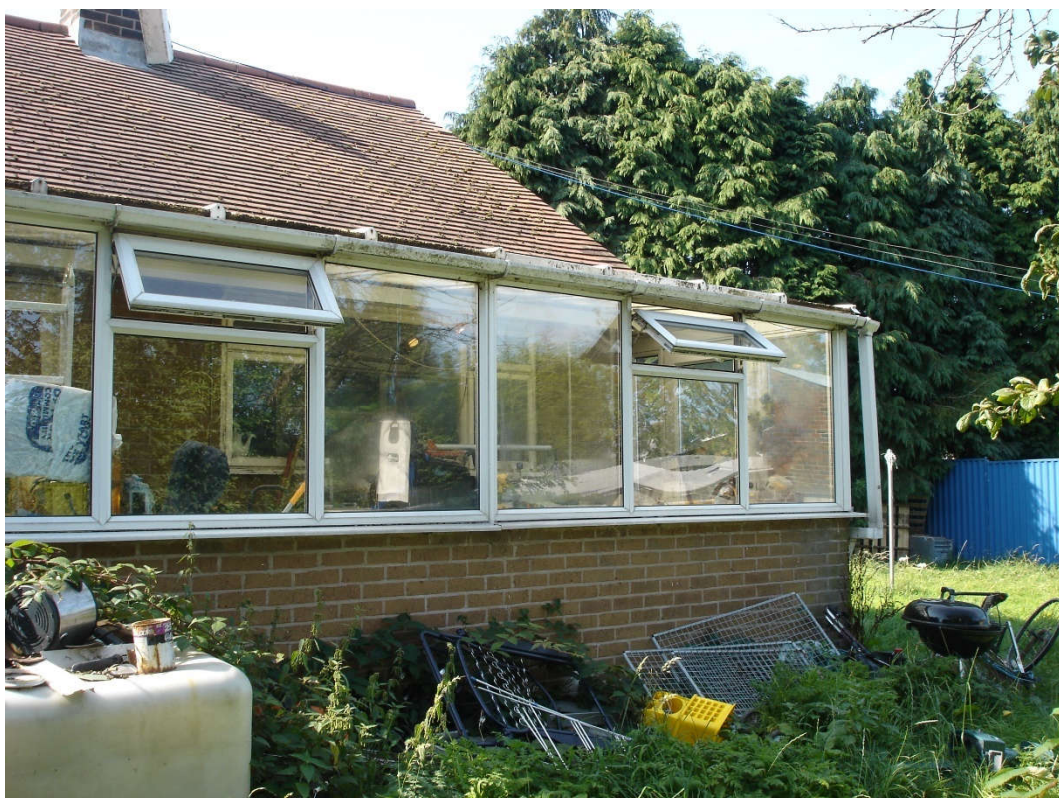
08. Rear conservatory – east elevation.
