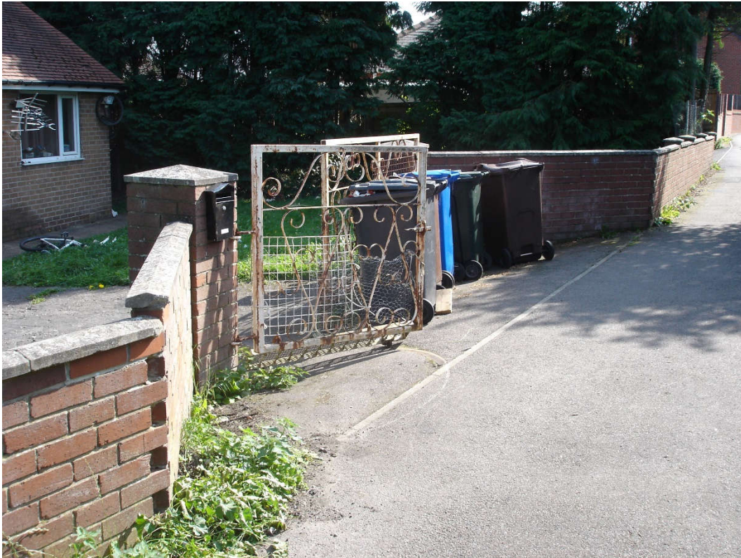
03. View of entrance to site from access lane.
