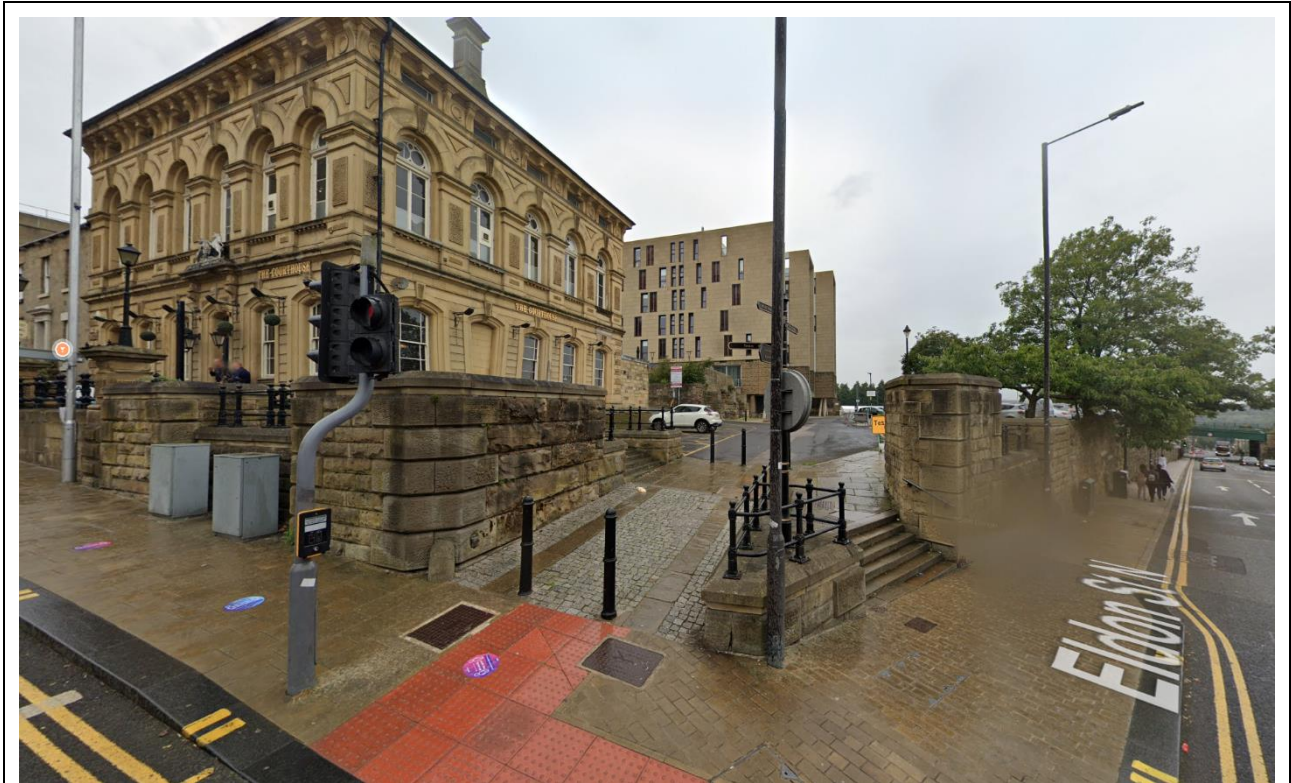
Figure 5.3: Existing pedestrian access off Regent Street / Eldon Street / Eldon Street North
