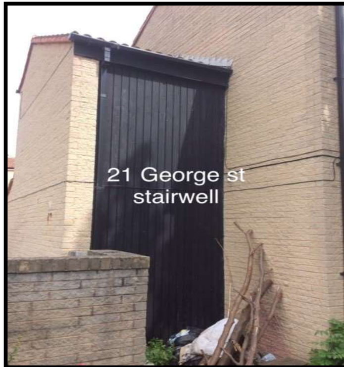
No. 21 George Street – Rear Elevation
