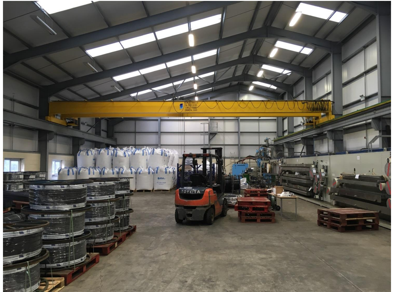
Inside the existing building
