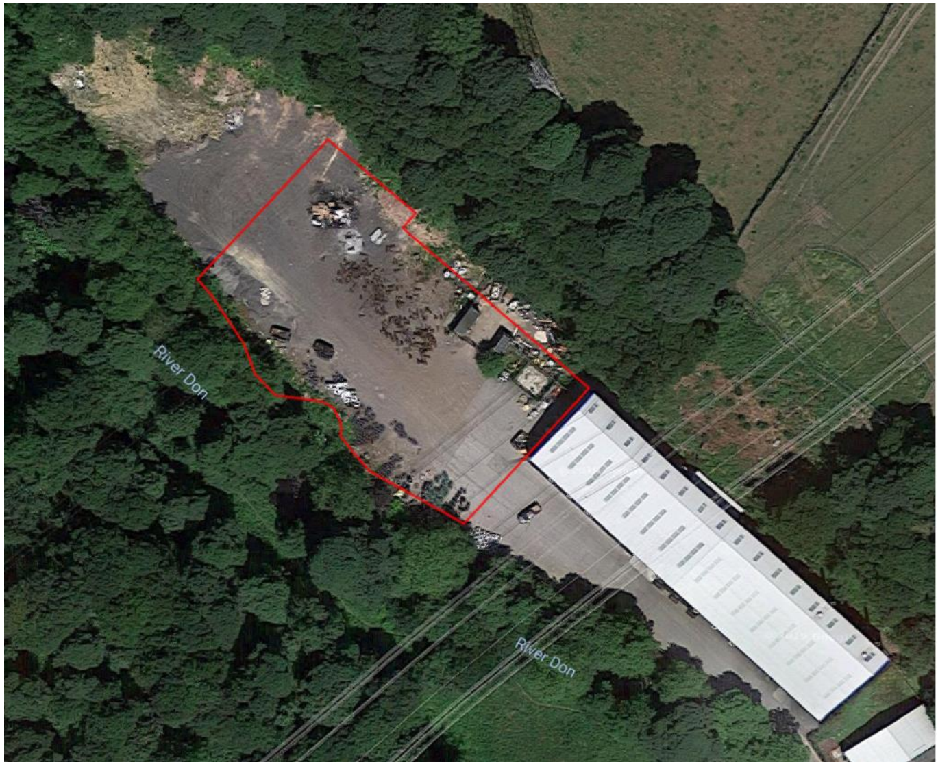
Extension to Existing Industrial Building
