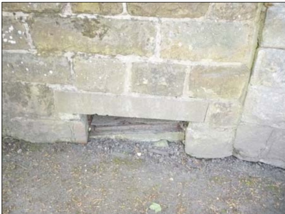
Title: GP33 Date: 14/5/18 Description: MANHOLE - UNDER WALL
