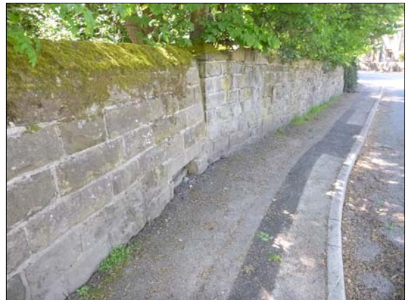
Title: GP34 Date: 14/5/18 Description: MANHOLE UNDER WALL - LOCATION
