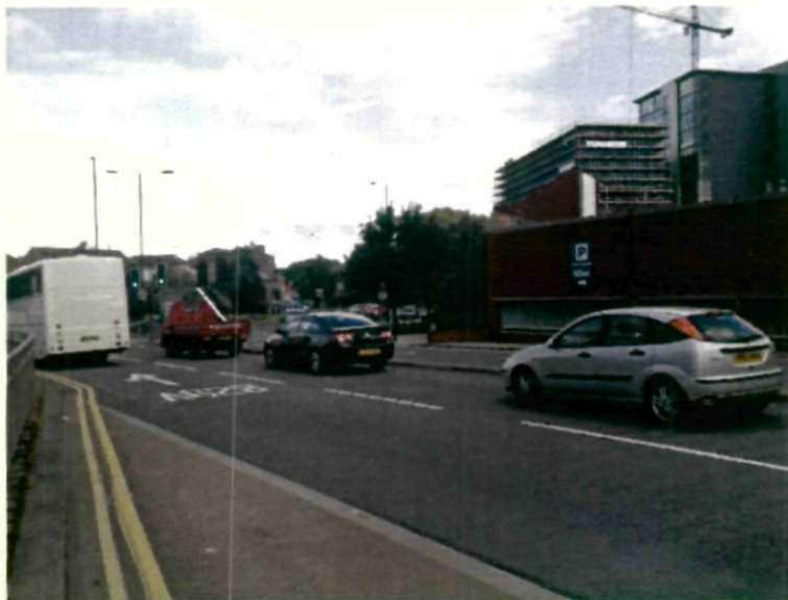
View North – West along West Way showing existing Supermarket and Gateway Plaza in distance – Highlights lack of integration between supermarket and highway
