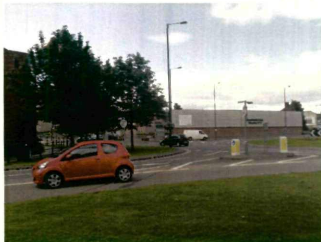
View South over roundabout towards Gaimster Quality – Highlights poor integration of building and roundabout
