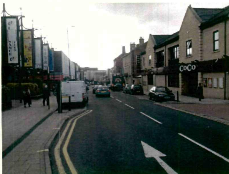
View East along Peel Street showing existing properties – Highlights poor integration of building styles and materials. Excessive signage.
