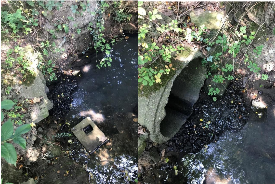
Photographs 1 and 2 indicating the pipe outfall located adjacent to Stead Lane
