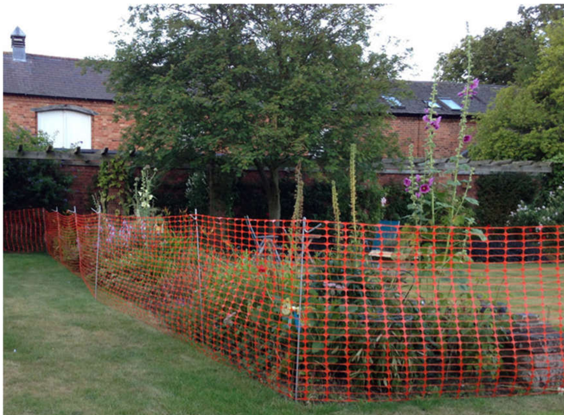
Figure 6: Plastic mesh fencing secured with heavy duty metal stakes
