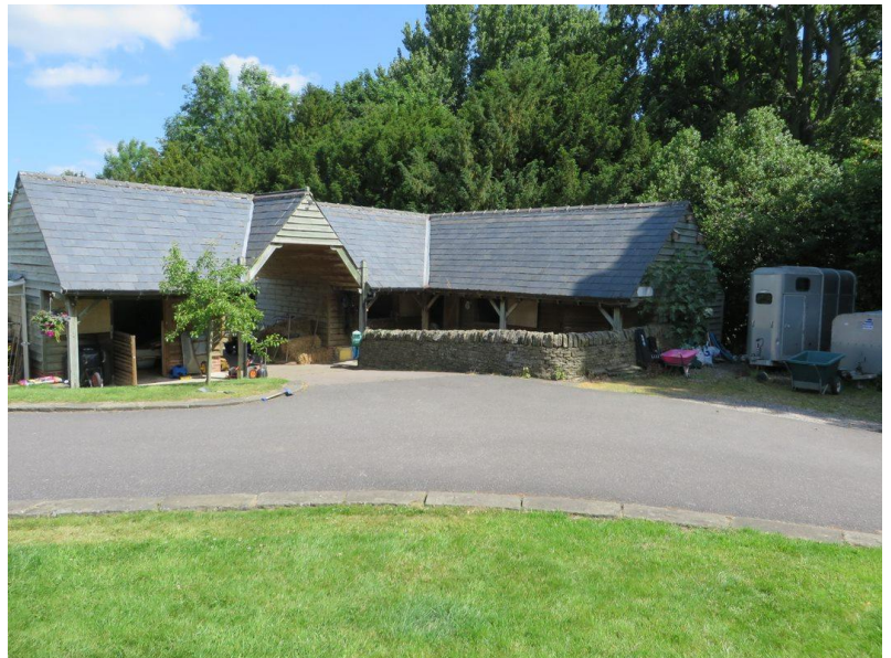
South Elevation of the barn
