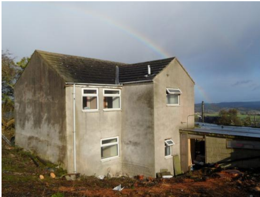
VIEW OF THE EXISTING HOUSE FROM THE REAR
