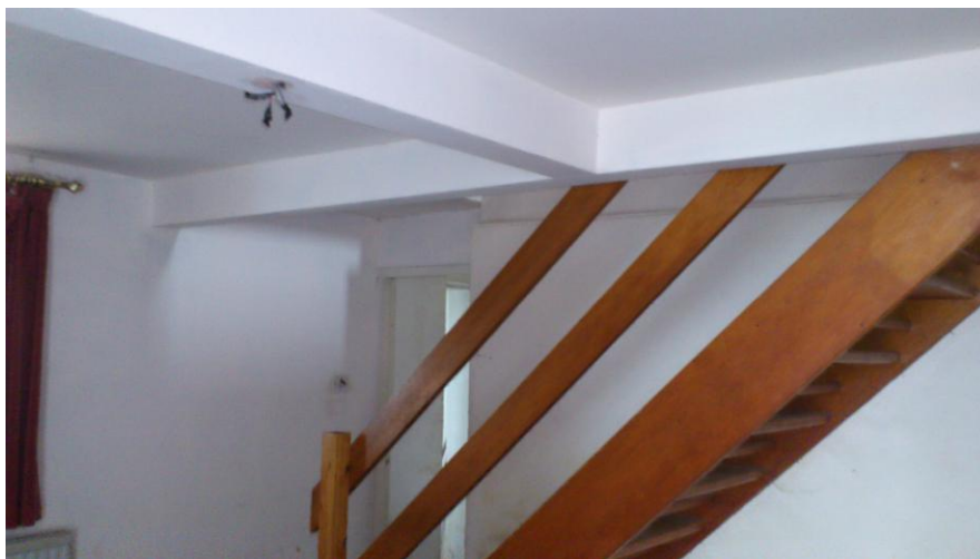
Internal stair with steel beams to ceiling
