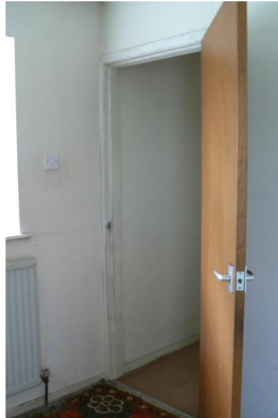
Typical internal door and frame with modern ironmongery. Small skirting and modern radiator
