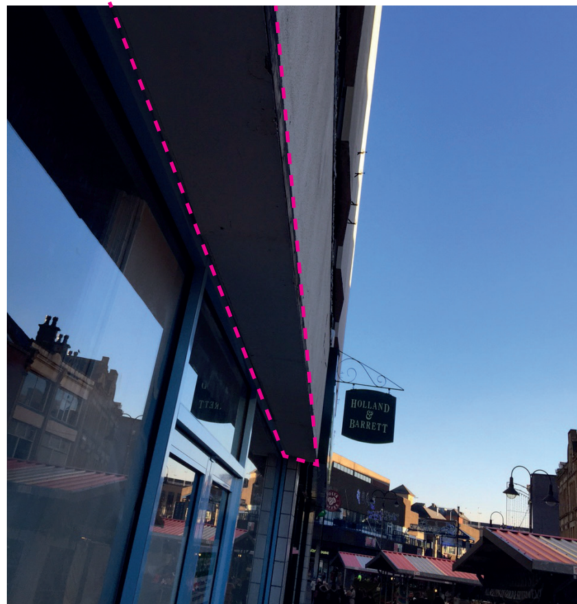
▲ Underside cladding panel location
