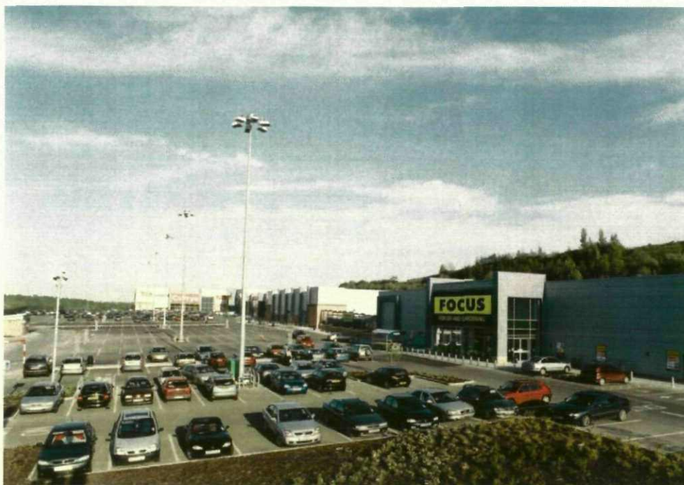
Fig. 1 View across existing car park – Unit 2 in foreground
