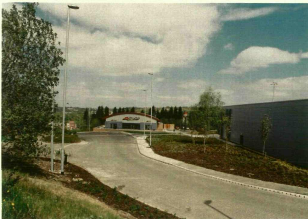
Fig. 2 View towards Pizza Hut – Unit 2 gable in foreground
