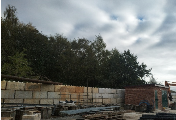
Photo 1: T1 and G2, looking southeast
