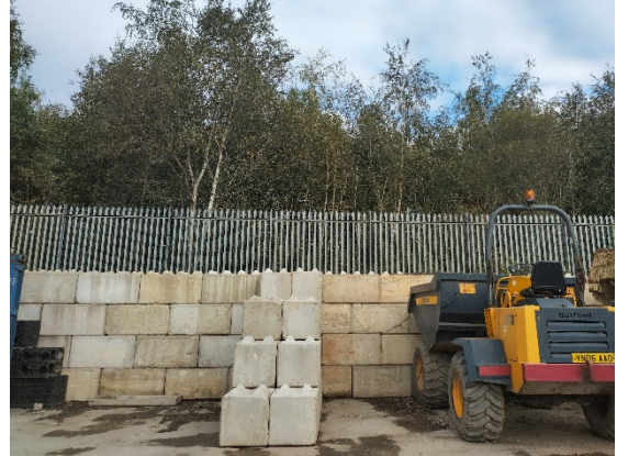
Photo 2: G2 looking east
