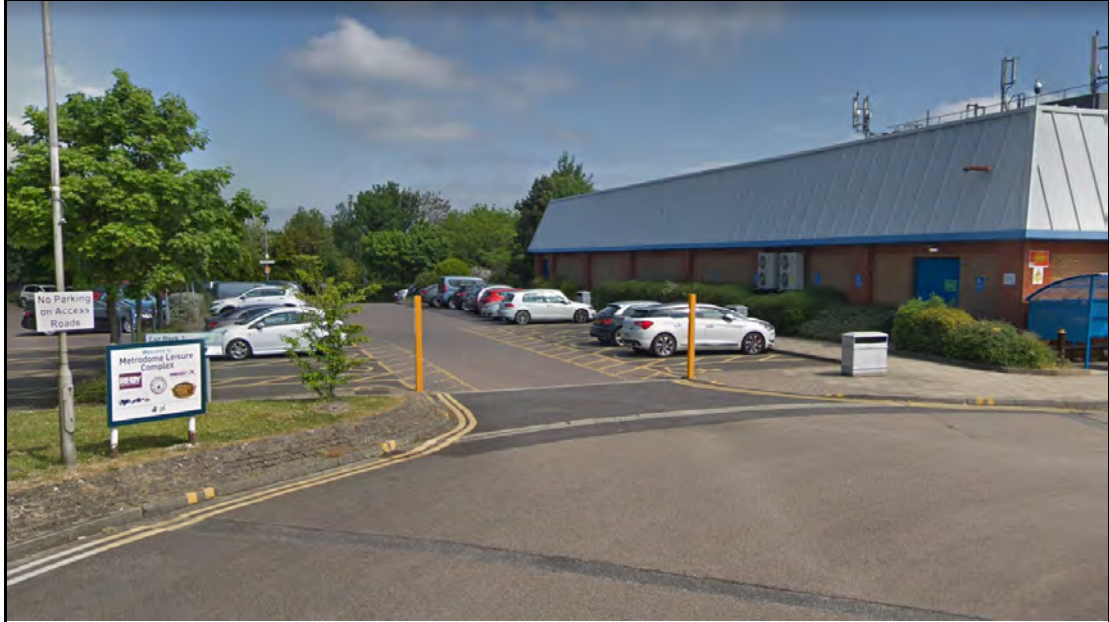
Figure 13: Existing Western Point of Access and Egress
