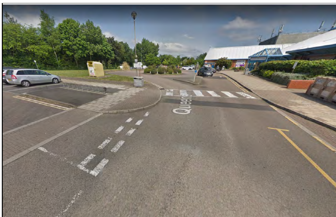
Figure 5: Footways and Crossings on Queens Road within site
