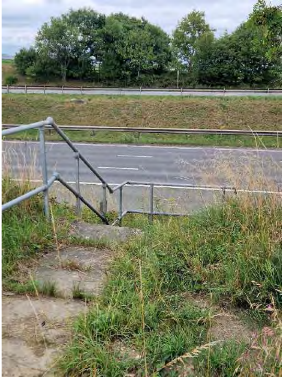
Site Photograph 4 - View to the East over the Highway Fenceline (North): A highway maintenance walkway and stairs was identified leading to the motorway. Note the horizontal platform prior to the cutting.
