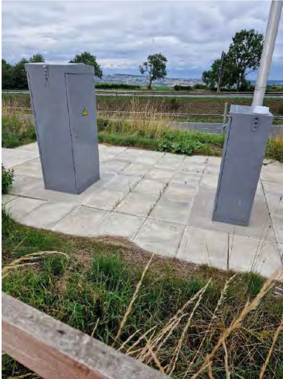
Site Photograph 5 - View to the East over the Highway Fenceline (South): A motorway communications installation was identified adjacent to the motorway. Note the horizontal platform of several metres prior to the cutting.
