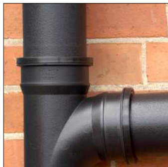
Black gutters and downpipes.
