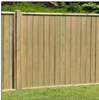
T & G vertical timber fencing.
