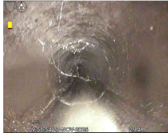
MH2X_5fe242ca-51cd-474f-ba45-63dcfa0048c7_20260313_11228_184.jpg, 00:00:18, 2.14 m Attached deposits, grease from 5 o'clock to 7 o'clock, 5% cross-sectional area loss, start
