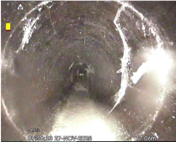
MH2X_6e421cfa-6512-4c62-974d-99e43f12887c_20260313_112330_536.jpg, 00:04:56, 17.06 m Roots, fine at joint
