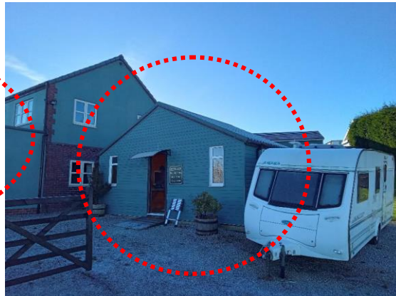
Single storey annex
