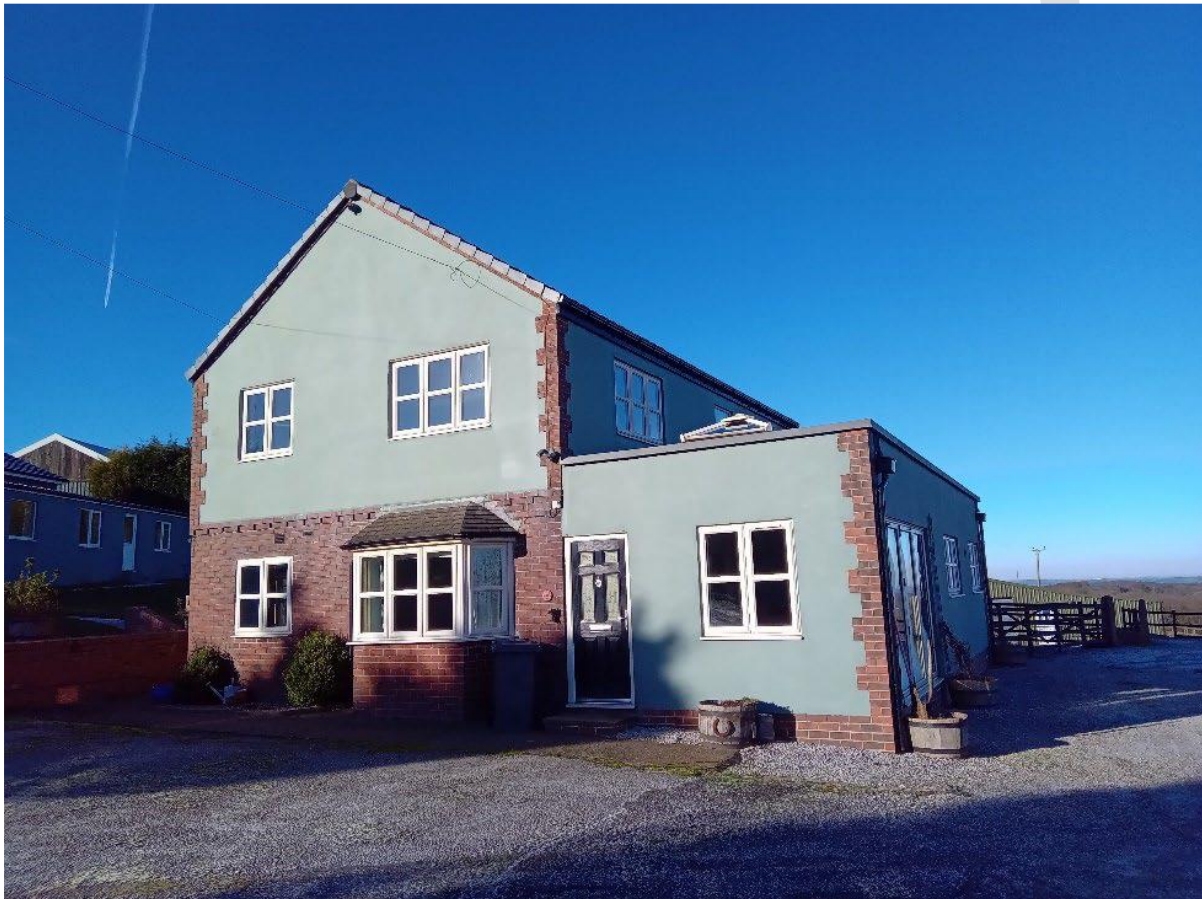
The existing detached house
