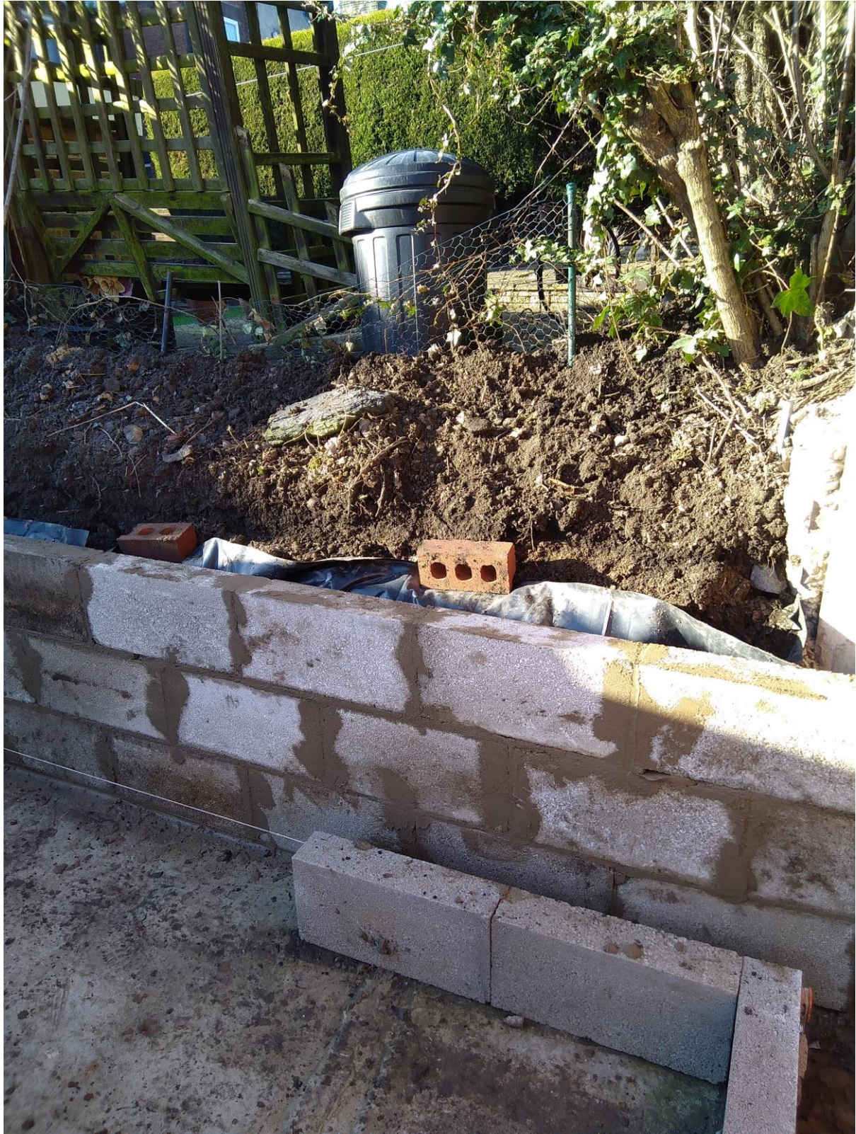
PHOTOGRAPH 10 SHOWS THE ONGOING WORKS TO THE EXTERNAL WALL OF THE BUILDING, ADJACENT TO THE EXISTING LAND, WITHIN THE CURTILAGE, WITH NO GAP. THE BLACK BIN THAT APPEARS IN MANY OF THE PHOTOS CAN CLEARLY BE SEEN. PHOTO No
