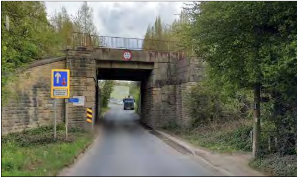
Figure 3-3 Shaw Lane Bridge Shuttle Working (Source: Google Maps)
