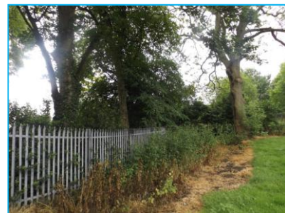
Figure 10 - Steel palisade fencing south of the car park
