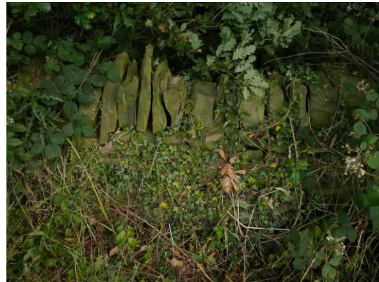
Plate 2: boundary wall along the eastern edge of site
