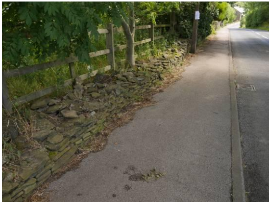
Plate 1: boundary wall seen from Cote Lane. Looking south
