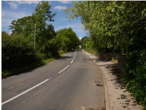
Plate 3: Access to the site from Cote Lane. Looking north
