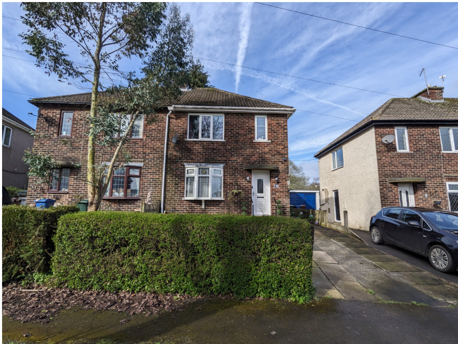
2209 - 10 West Crescent, Oxspring Front (East) elevation viewed from West Crescent
