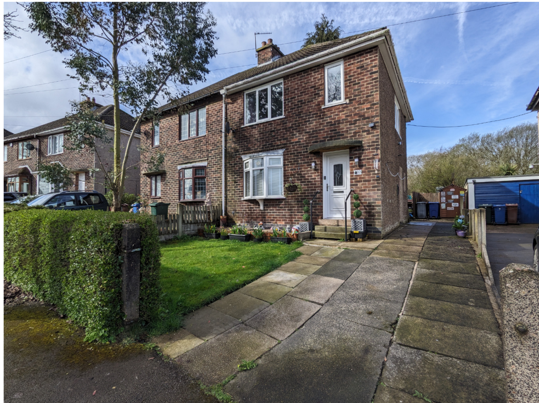
2209 - 10 West Crescent, Oxspring Front (NE) elevation viewed from West Crescent
