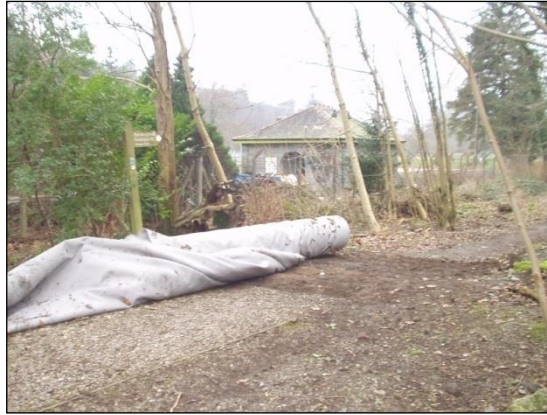
Photo 2- laying of Fibretex material onto existing subgrade.
