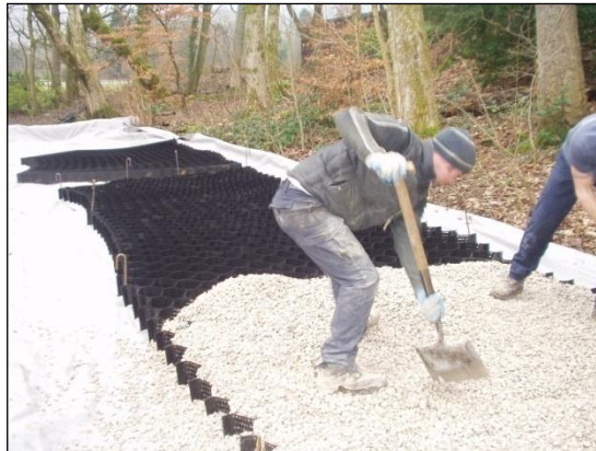
Photo 3- expanding and filling the Cellweb system
