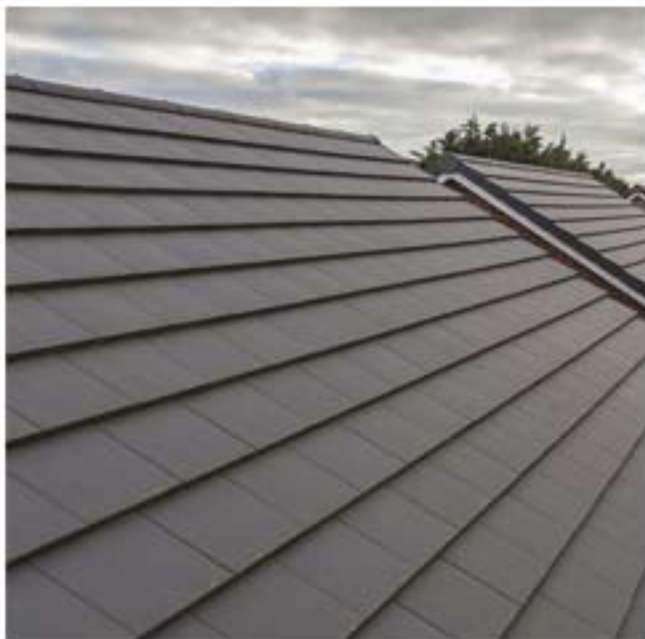
Marley Modern grey interlocking concrete roof tiles
