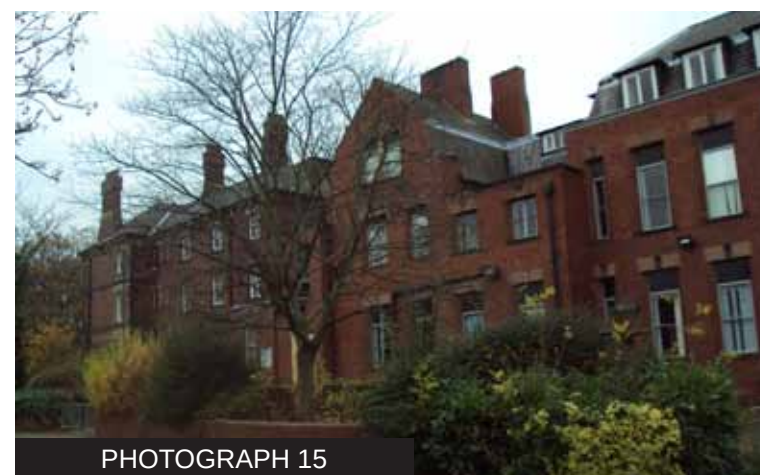
The rear of the Edwardian Villa (LH side) from Berneslai Close showing how the later extension joins unsympathetically to it.
