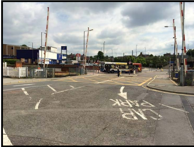
Photograph 2 – Existing Kendray Street level crossing
