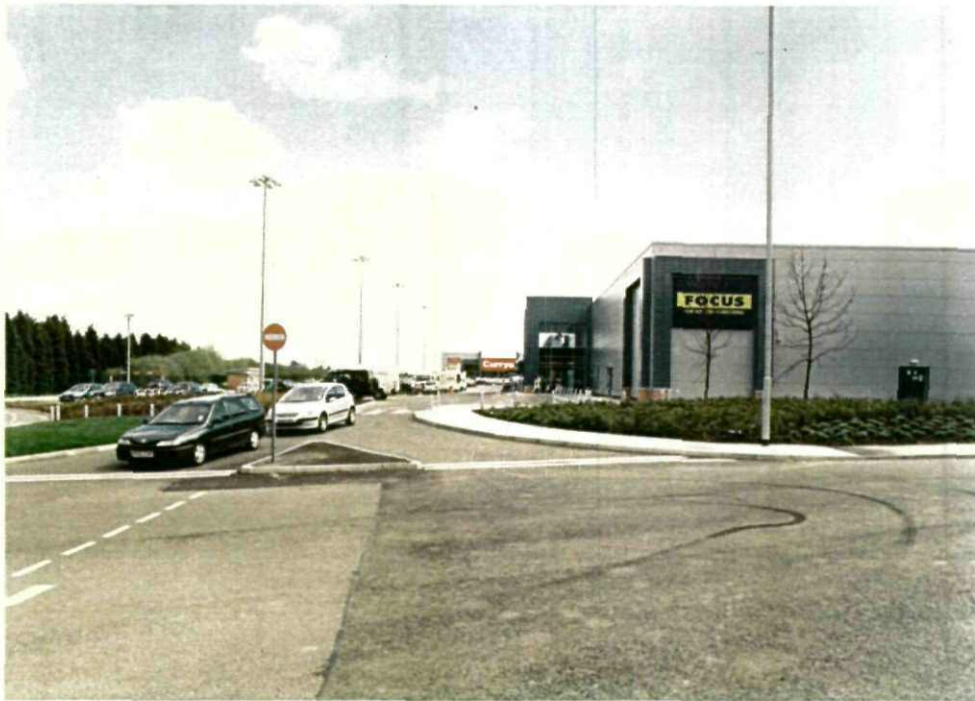
Fig. 3 View towards entrance of Focus DIY
