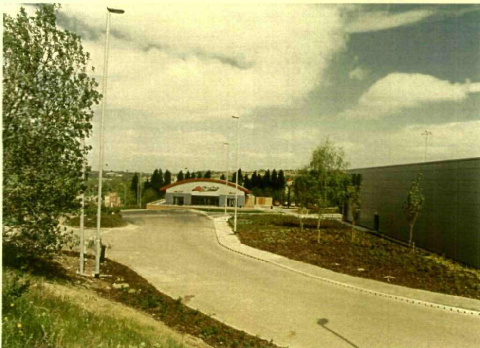
Fig. 2 View towards Pizza Hut – Unit 2 gable in foreground
