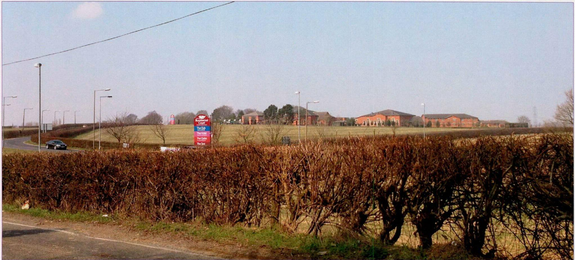
⑱ View of Burntwood Court from Common Road leading to South Kirkby.
