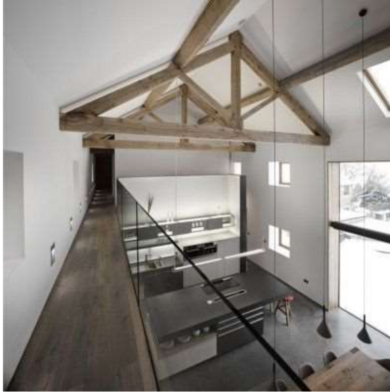
Fig. 05. The intention is to retain the central threshing floor of the barn open and without sub-division.
