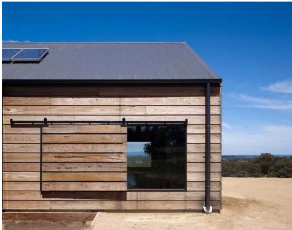
Fig. 01. Sliding timber shutters, timber cladding and a profiled metal roof reference other modern agricultural buildings in the area.
