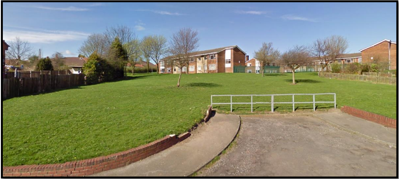
The photograph above shows the current access to the site; with the now demolished Sandhill Court Sheltered Housing complex in the background.
