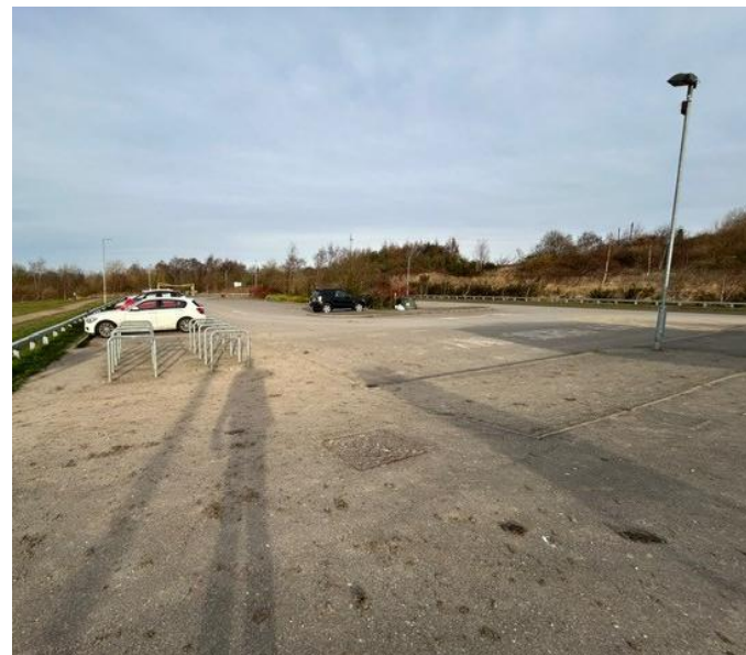
Existing Car Park looking north-east
