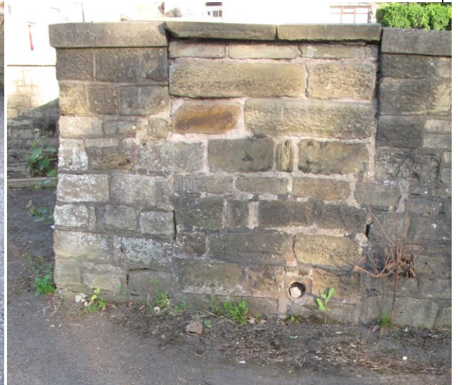
Barnsley Road side of boundary wall showing gully outlet pipe
