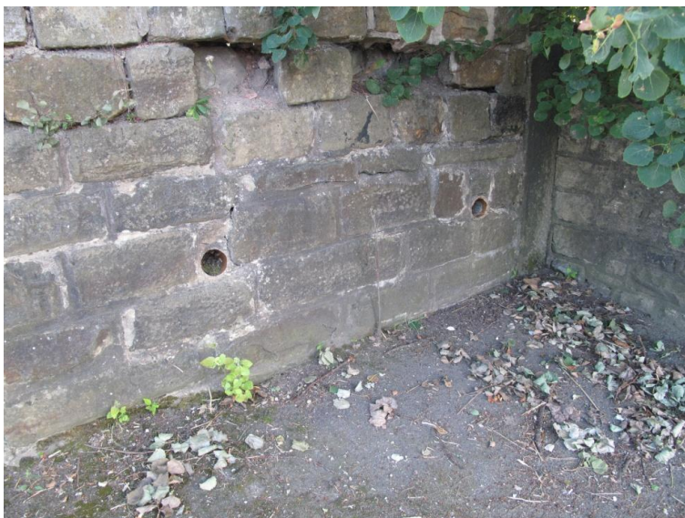
Weep holes in boundary wall
