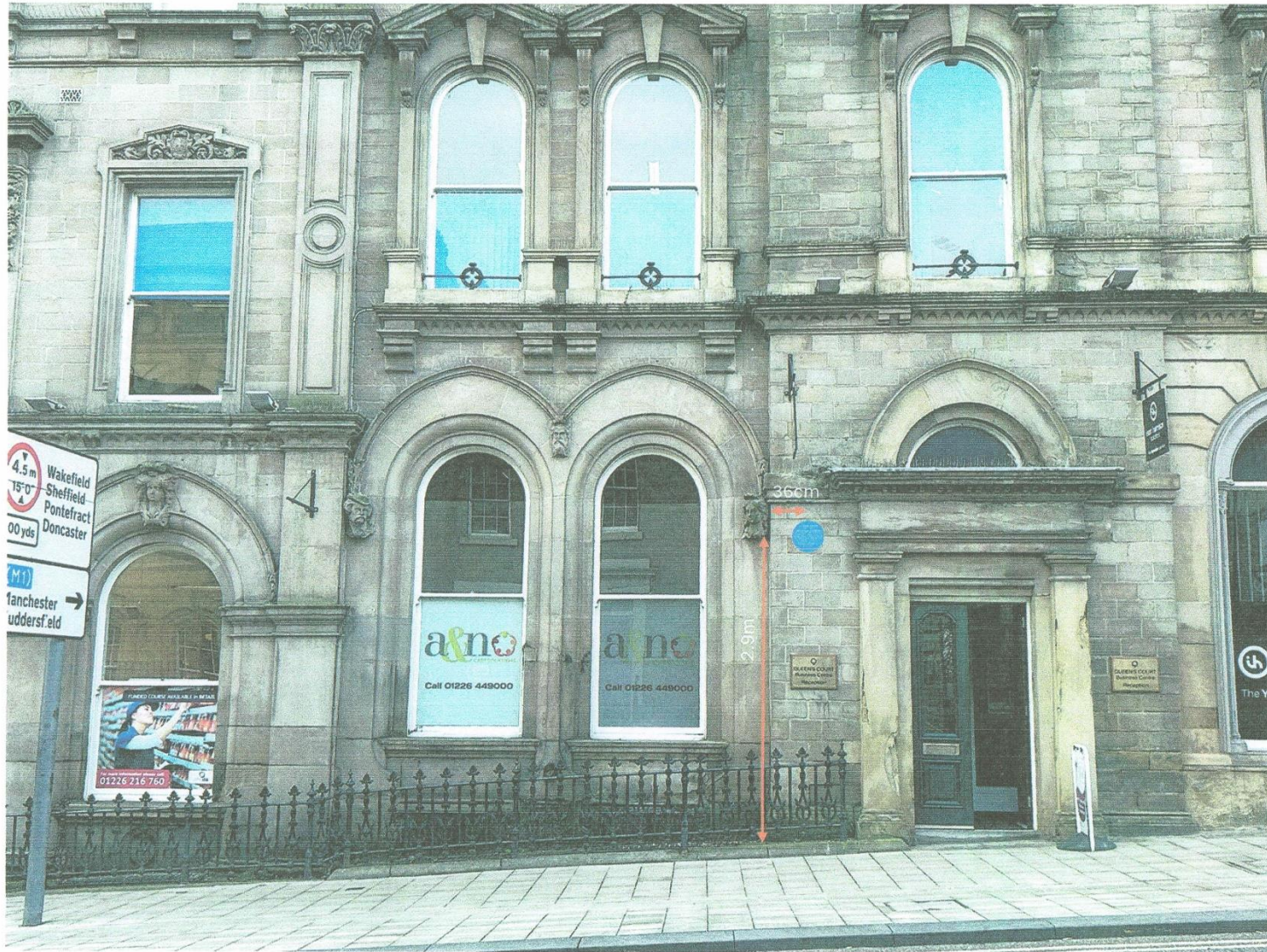
Queen's Court Business Centre (Queen's Hotel) Front Elevation showing proposed position of Blue Plaue
