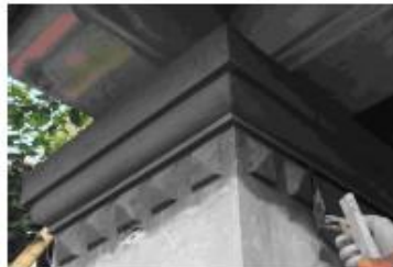
IMAGE 2 - INDICATIVE IMAGE OF K REND DETAILED Moulding (REFER TO PROFILE DETAILS). COLOUR TO BE SANDSTONE (NOT CHARCOAL AS ILLUSTRATED).
