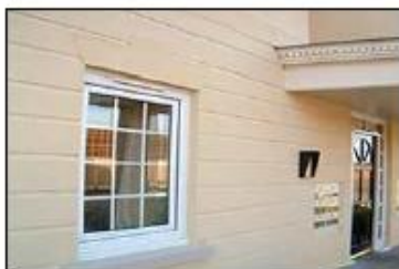
IMAGE 1 - INDICATIVE IMAGE OF K REND ASHLAR TOOLED FINISH (REFER TO DETAIL). COLOUR TO BE SANDSTONE (NOT CREAM AS ILLUSTRATED).
