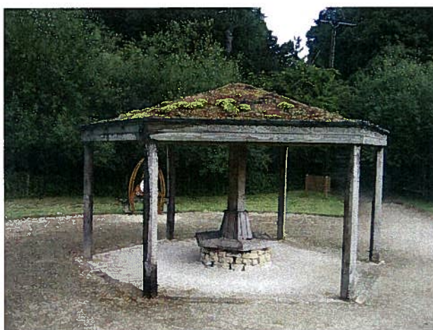
Shelter with Sedum Roof
