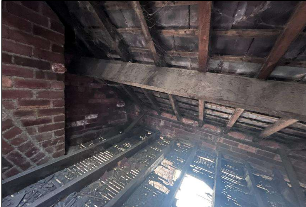
Plate 5. The roof void prior to reroofing
