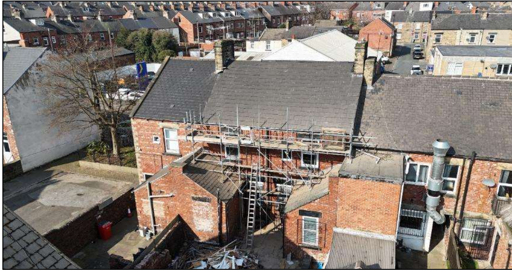
Plate 3. The rear of the building (viewed from the southeast)
