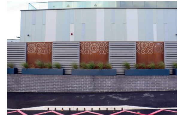
Laser-cut weathering steel panels screening The Memorial Garden at The Luton and Dunstable Hospital, Lewsey Road, Luton.
