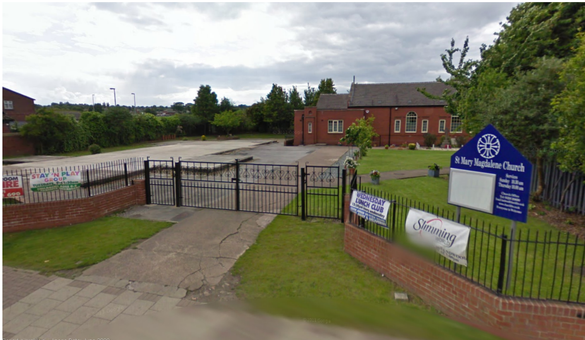
729002352 – Street View - Proposed Site for Activity Room for the Parish Church of St Mary Magdalene
