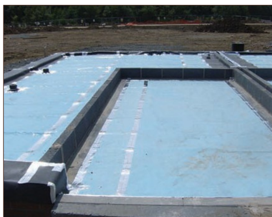
Figure A4.10 Almost complete coverage available for inspection, minimal jointing, service entries suitable distance from walls, light traffic (courtesy Smith Grant)
