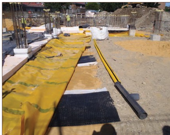
Figure A4.8 Geovent beneath the 2000g taped gas membrane lined up with collector pipes (courtesy Alderburgh Group)
