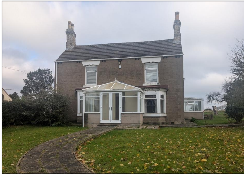
Plate 15. Looking northeast at the farmhouse principal elevation
