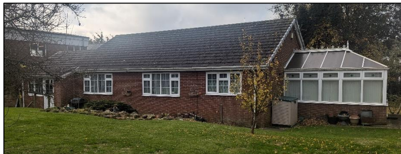
Plate 21. Looking south at the rear elevation of the bungalow
