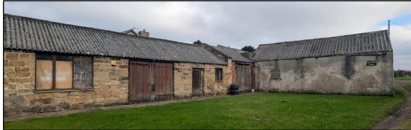
Plate 17. Looking north at the block of outbuildings
