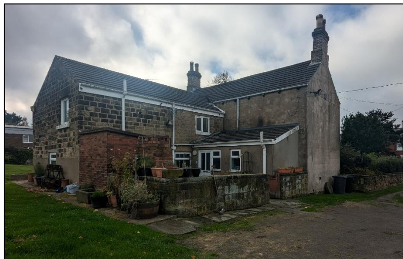
Plate 16. Looking south at the rear elevation of the farmhouse
