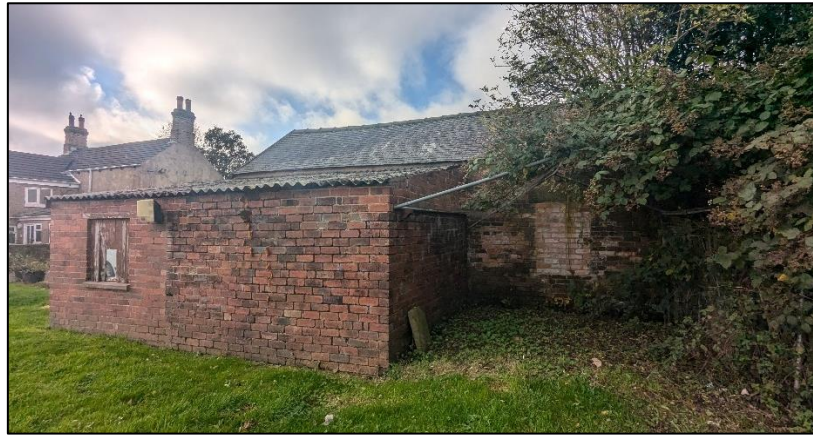
Plate 19. Looking southwest at the block of outbuildings
