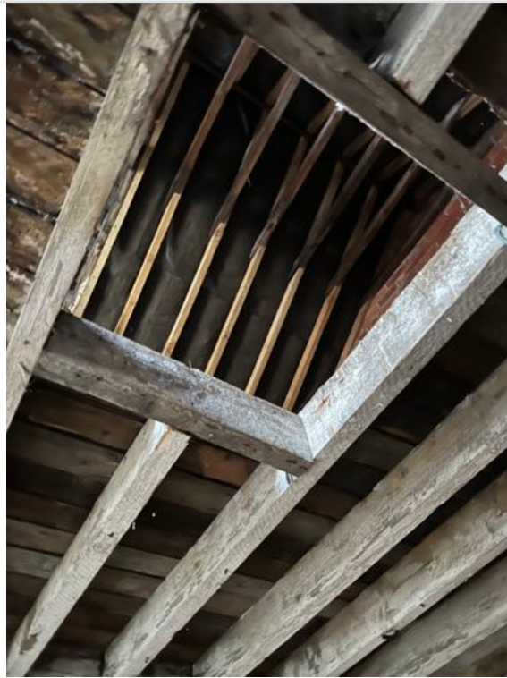
Photo 12 - Underside of first floor with felted roof above.
