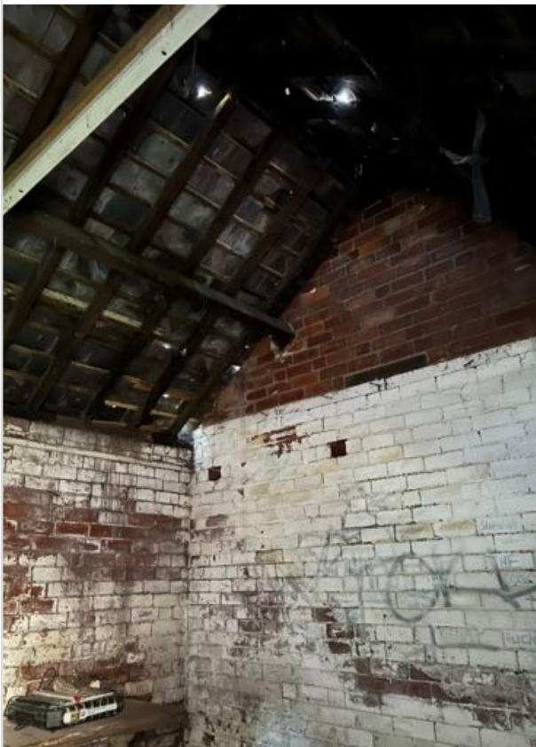
Photo 9 - Roof Space - Single Storey
