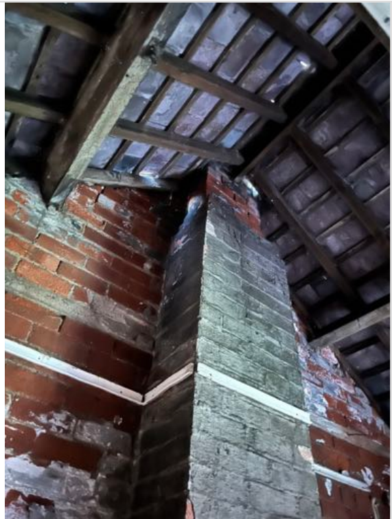
Photo 8 - Roof Space - Single Storey
