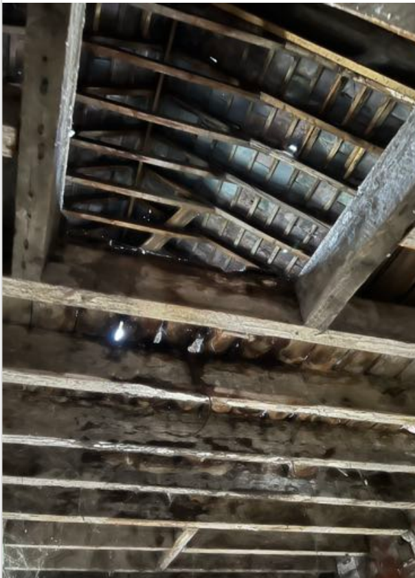
Photo 14 - Underside of first floor with exposed roof structure above.
