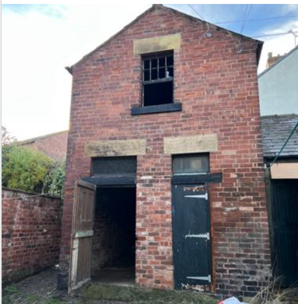
Photo 5 - Front Elevation - 2 Storey
