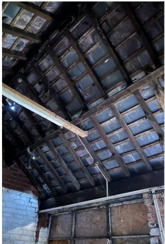
Photo 10 - Roof Space - Single Storey
