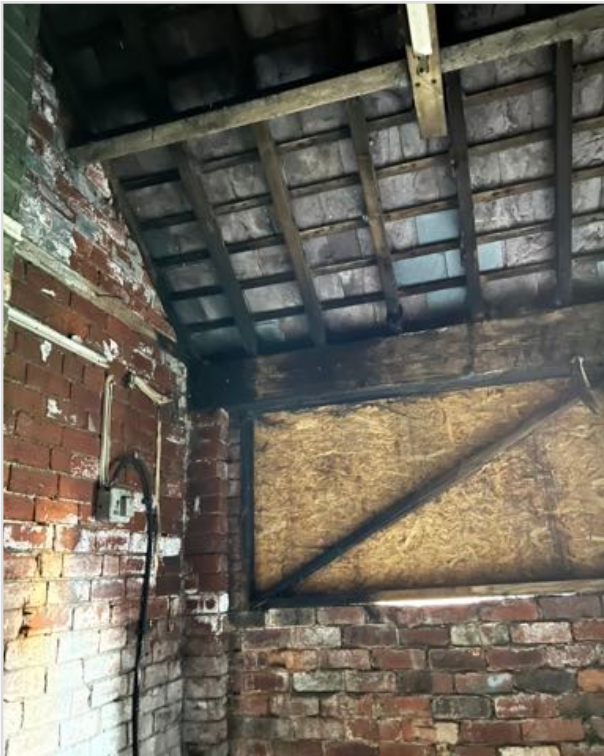
Photo 7 - Roof Space - Single Storey
