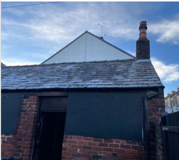
Photo 3 - Front Elevation - Single Storey
