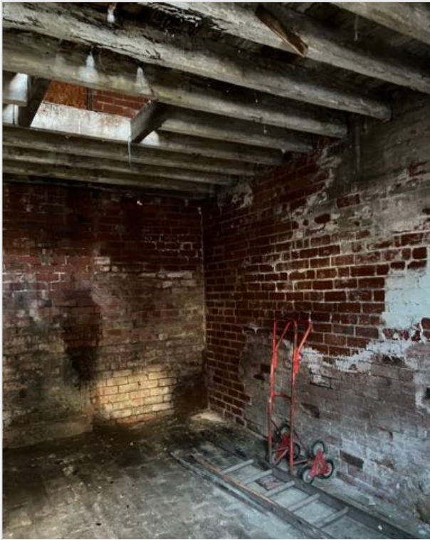
Photo 11 - Underside of First Floor
