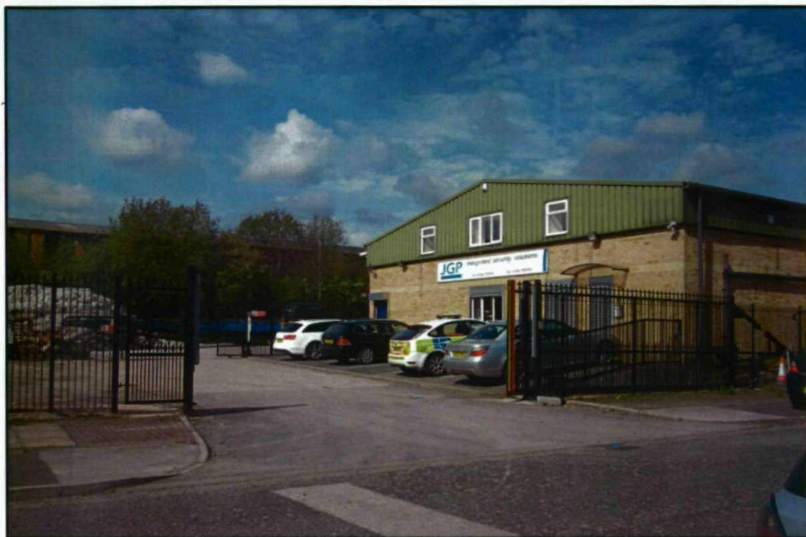
Photograph 2 View of site building with gated entrance to car park and yard beyond.
