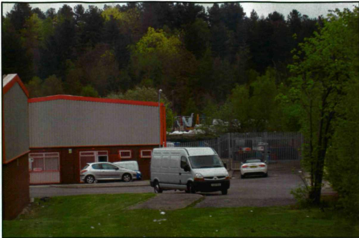
Photograph 19 Industrial premises to south-west of site, partially on infilled canal.
