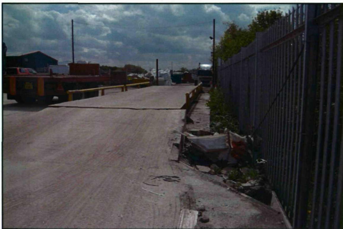
Photograph 14 View of weighbridge along south-western boundary.
