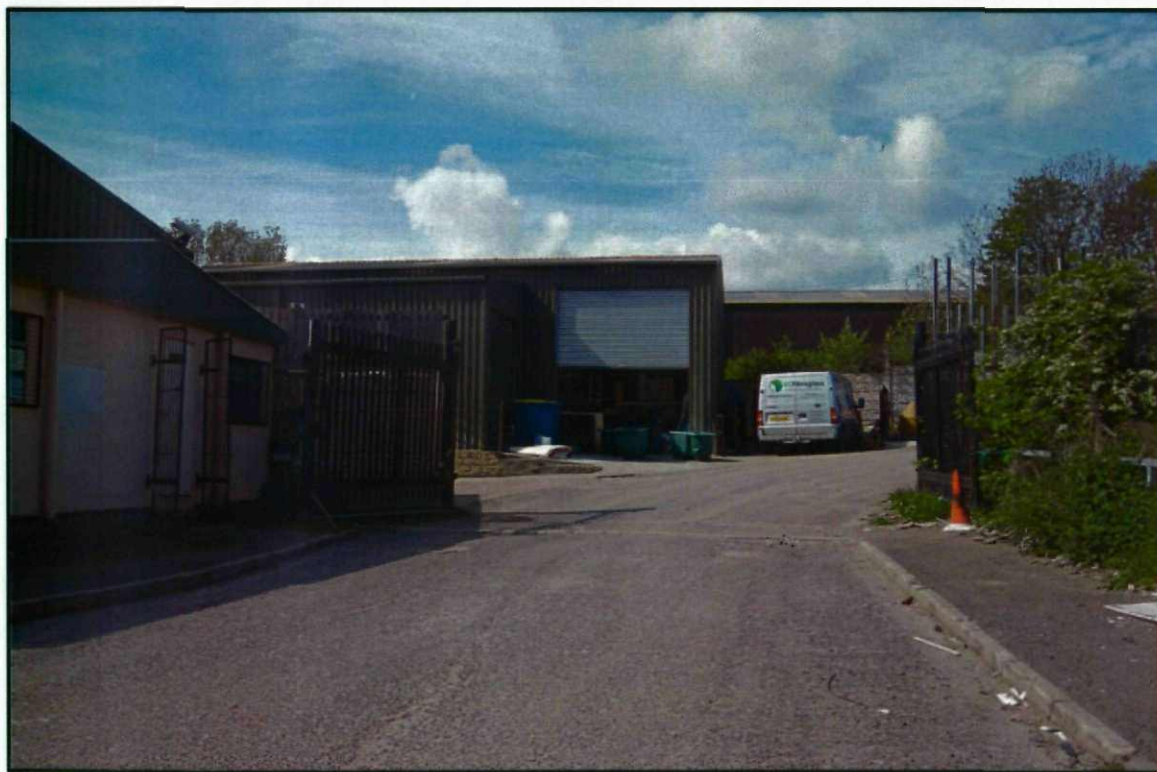
Photograph 4 Entrance to northern yard.
