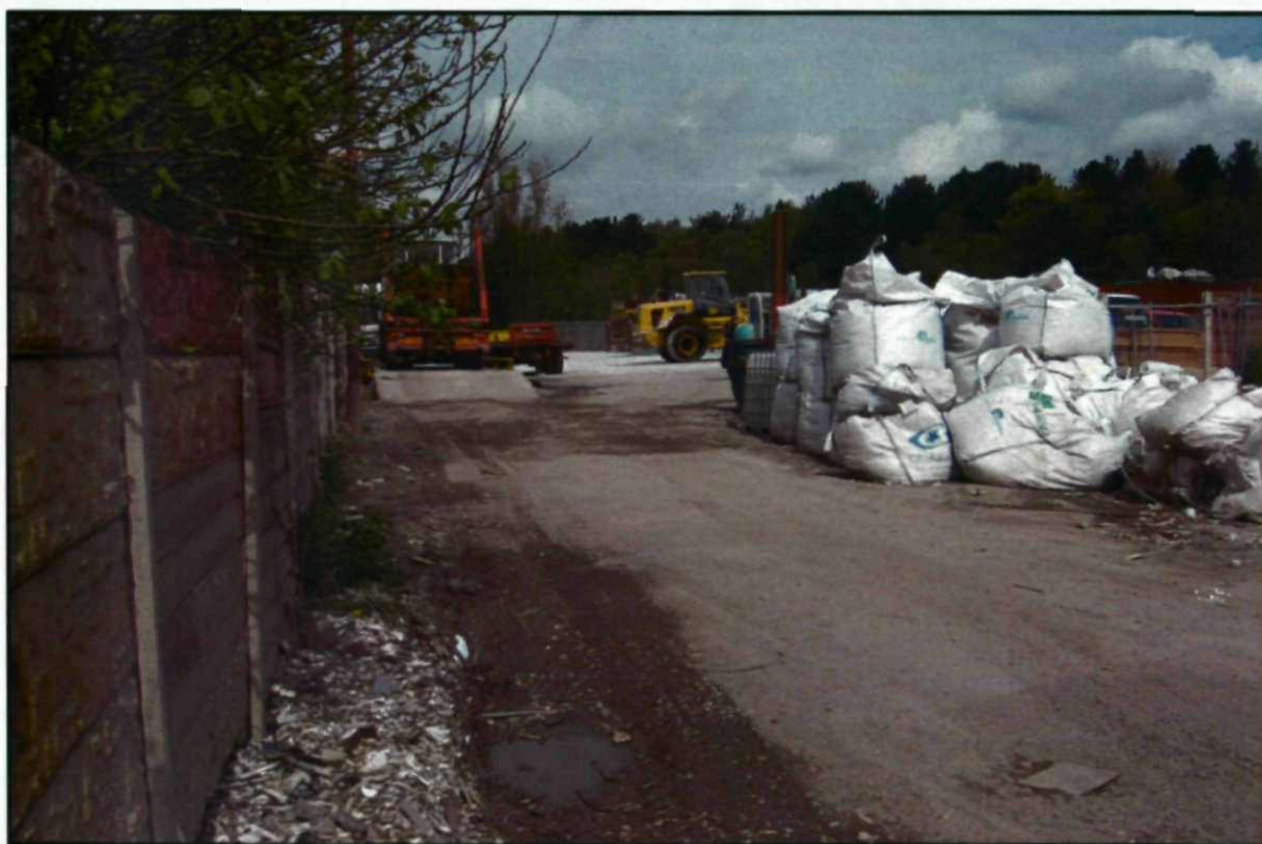
Photograph 8 Access point between two parts of northern yard.
