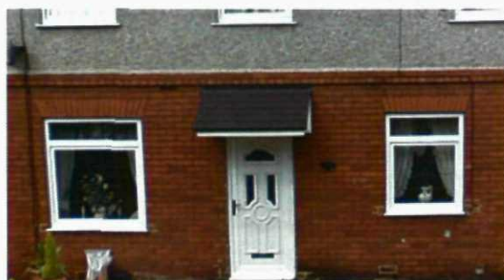
Architectural detailing along Higham Lane
