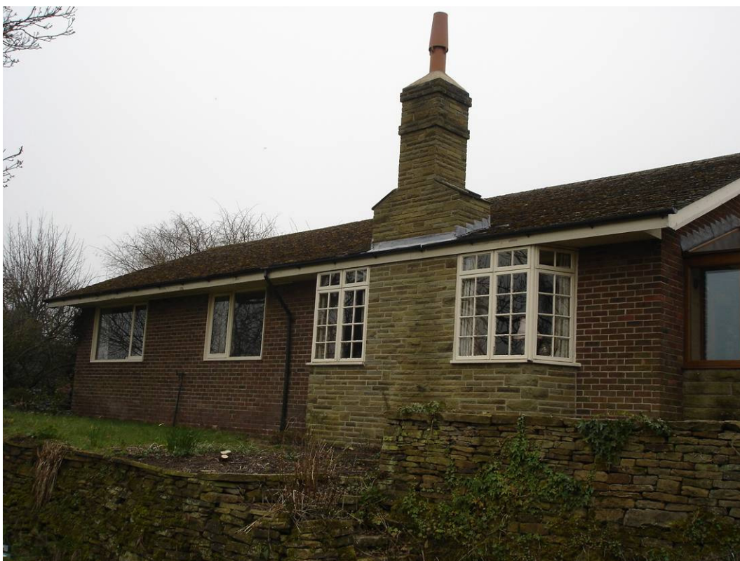
0.5 North elevation of bungalow.
