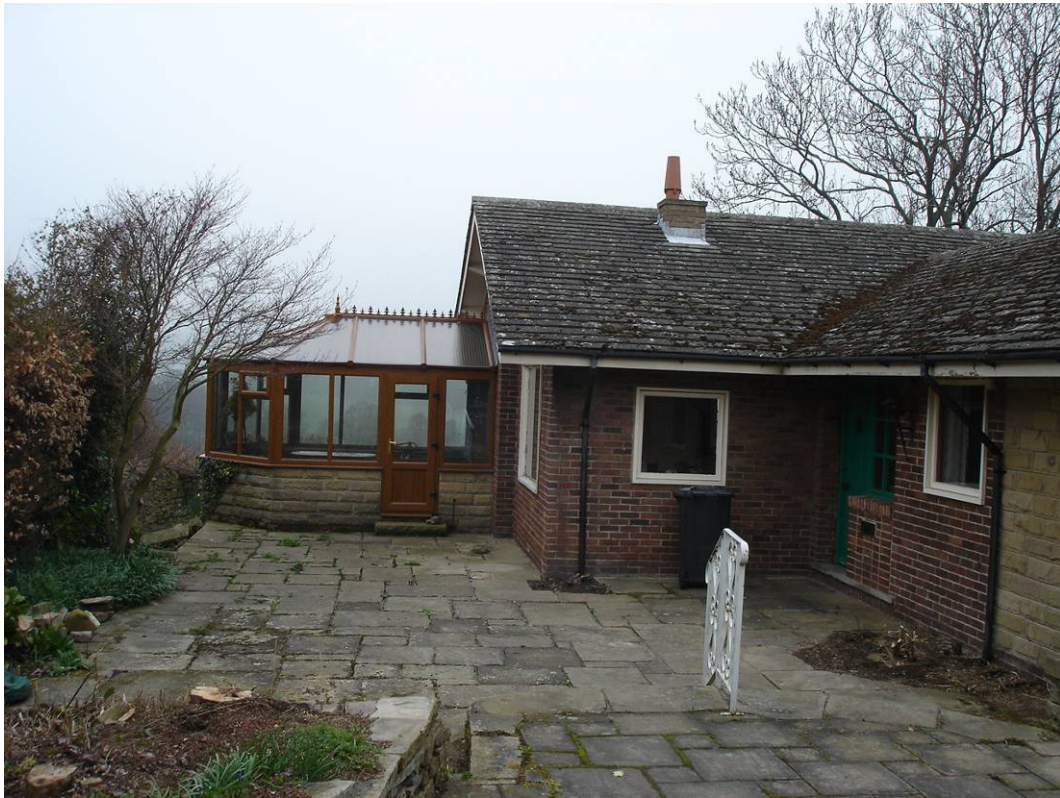
0.3 View from parking area looking North.
