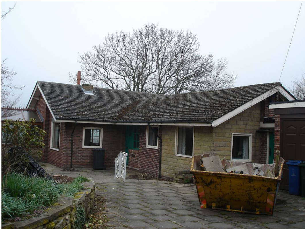
0.2 View of bungalow from access gate.
