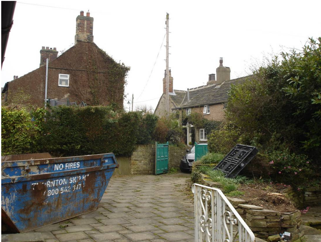
0.7 Existing parking and adjacent dwelling to Cliffe Hill.
