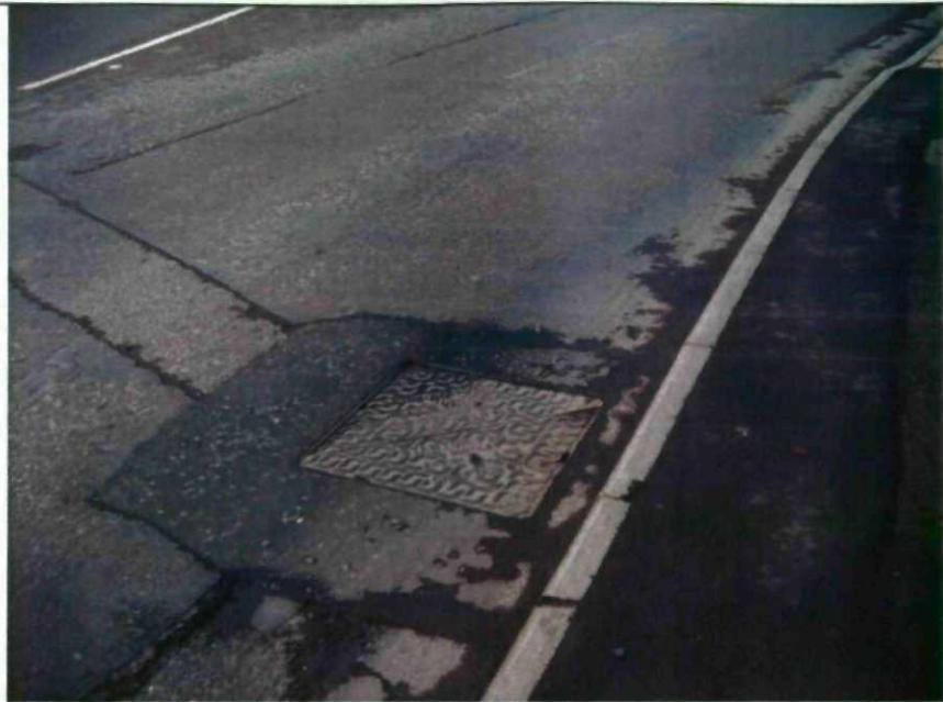
Photograph 13 – Outside the north west boundary of the site on Burton Road was a manhole which indicates existing drainage channels.
