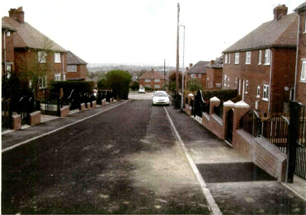
View looking down Vernon Close at the recent environmental works.
