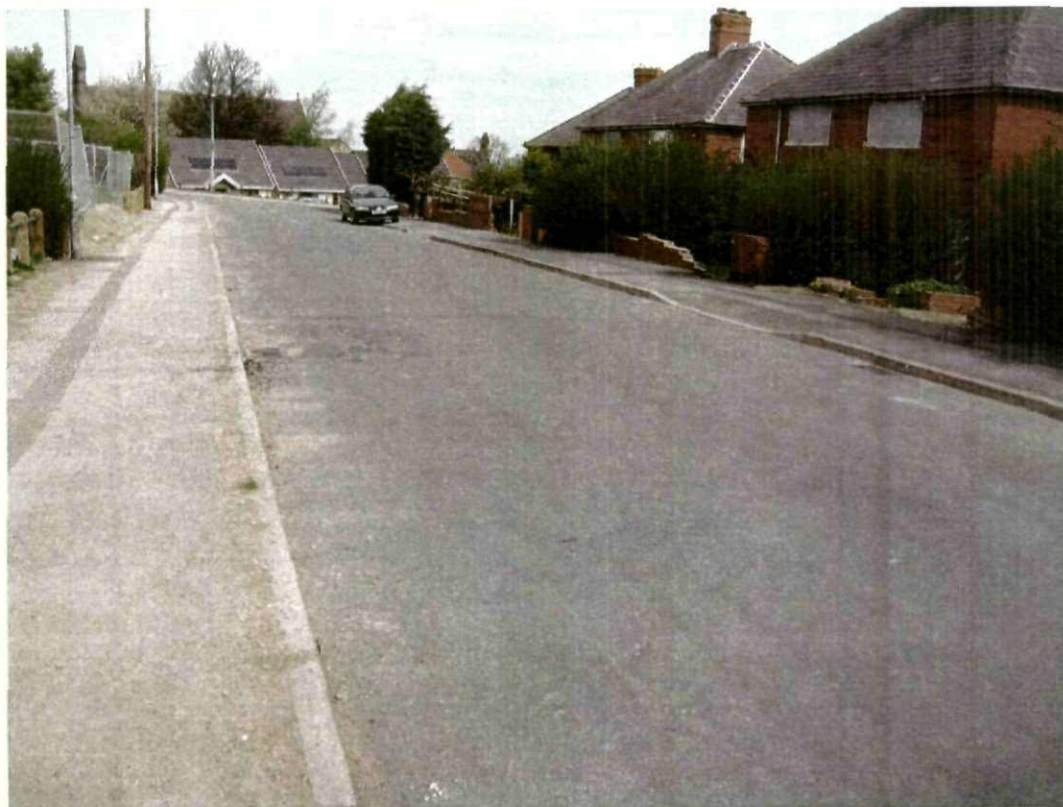
View along top of Bruce Avenue towards Mount Vernon Avenue with Phase 1 bungalows in the distance and Phase 2 to the left.
