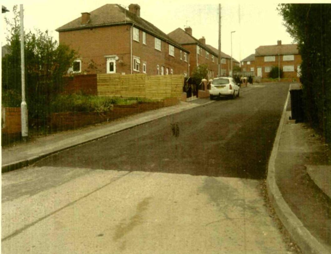
View looking east up Vernon Close towards the new environmental works.
