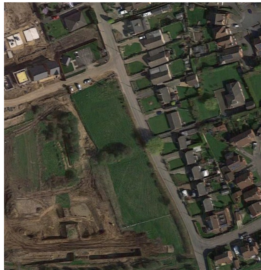
Figure 3- Aerial View of existing site
