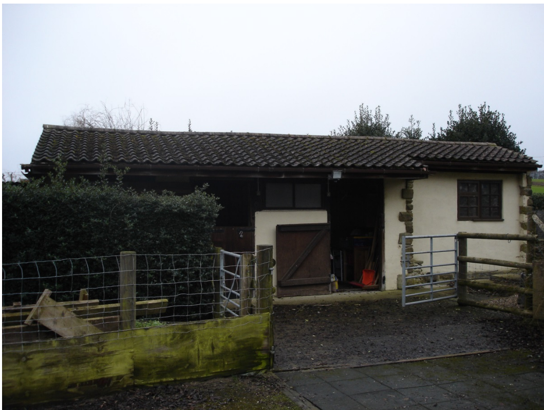
Fig 1. Existing building viewed from frontage
